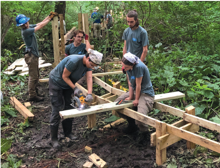
Previous page: The CFPA Summer Trails Crew poses on the timber crib steps they built at their Goodwin Conservation and Education Center. Left: Molly Bernstein sets rocks in a causeway to reduce erosion on the Charles L. Pack Trail at People’s State Forest. Right: The Trails Crew constructs an elevated bog bridge at Timberland Park in Berlin.
