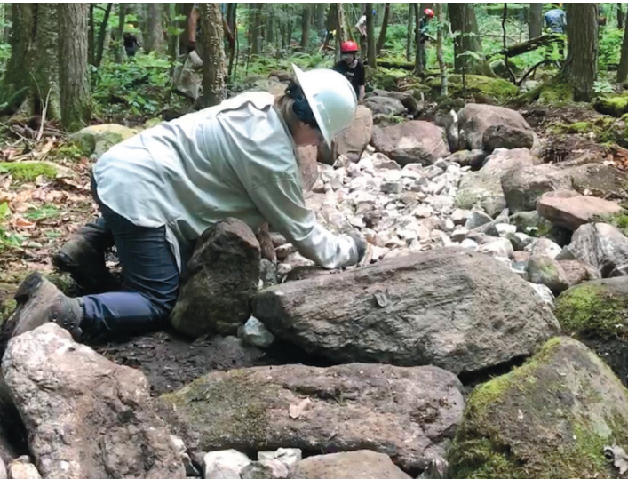
Previous page: The CFPA Summer Trails Crew poses on the timber crib steps they built at their Goodwin Conservation and Education Center. Left: Molly Bernstein sets rocks in a causeway to reduce erosion on the Charles L. Pack Trail at People’s State Forest. Right: The Trails Crew constructs an elevated bog bridge at Timberland Park in Berlin.
