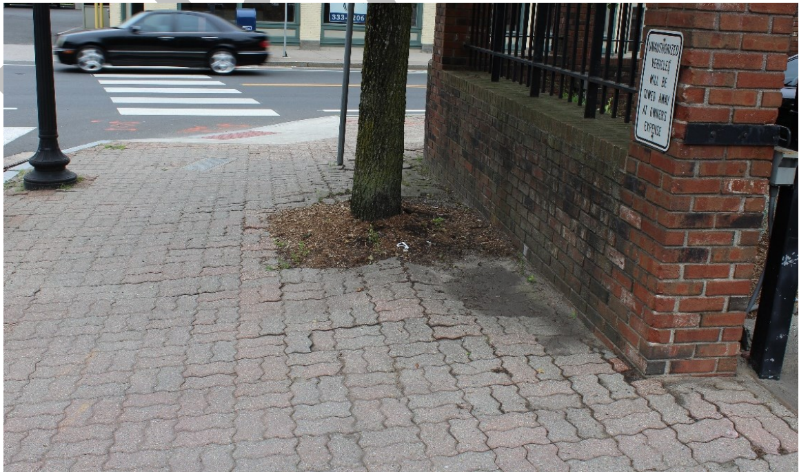
Heaving Sidewalk on Washington Street
