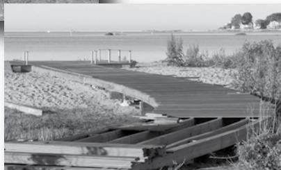
Installation of Diamond Pier foundations at Chittenden trailhead—shown are siting of piers (top left), closeup of single pier (middle); installation of boardwalk over framing (bottom right); two piers supporting framing (center). All photos provided courtesy of Steve McGuire.
