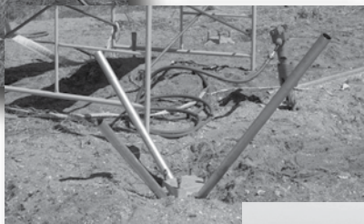
Installation of Diamond Pier foundations at Chittenden trailhead—shown are siting of piers (top left), closeup of single pier (middle); installation of boardwalk over framing (bottom right); two piers supporting framing (center). All photos provided courtesy of Steve McGuire.
