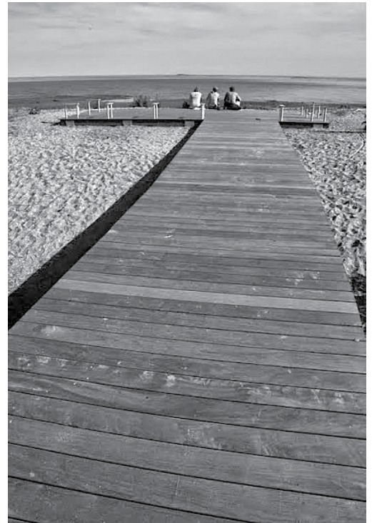
This page: The decking and benches are made of rot- and salt-resistant Ipe wood.
