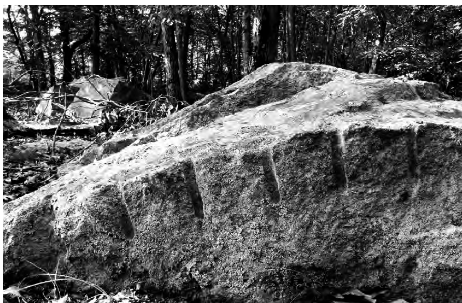
Stonecutter's holes, shown here in cross section, made way for feathering wedges.
