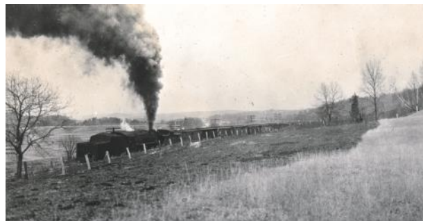
Strip along railroad burned as a precaution against forest fire. Source: Connecticut Forestry Department
